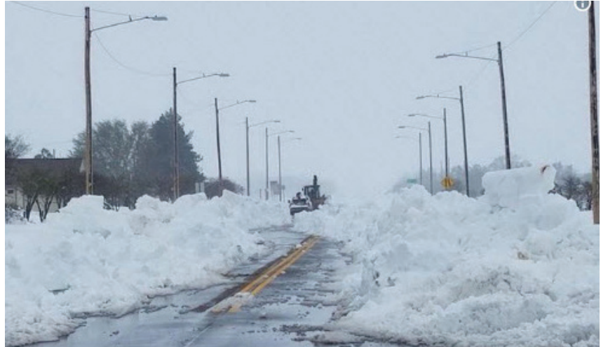
Crews work to remove snow and re-open roads in the City of Lakin after last year's spring blizzard.
